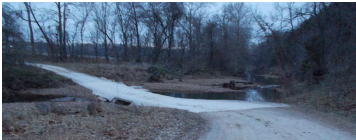
Ellis Davis Road Bridge, Cooper County, Missouri Old low water crossing and new bridge
