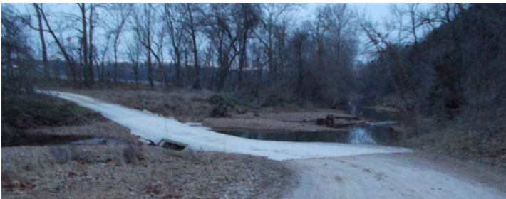
Ellis Davis Road Bridge, Cooper County, Missouri Old low water crossing and new bridge
