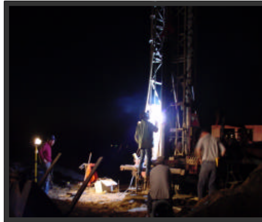
Drilling contractor working through the night
