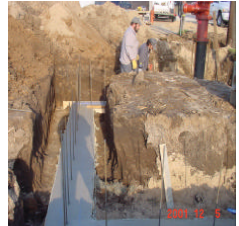
Poured footings for the New Control Building
