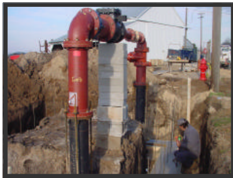
Piping for the new wells in the control building
