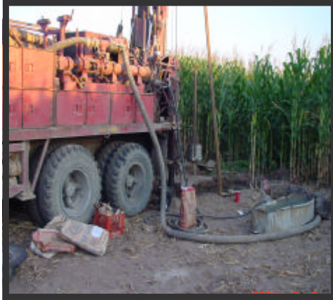
Drill Rig set-up and ready to start drilling operations
