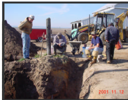
City crews completing piping connections
