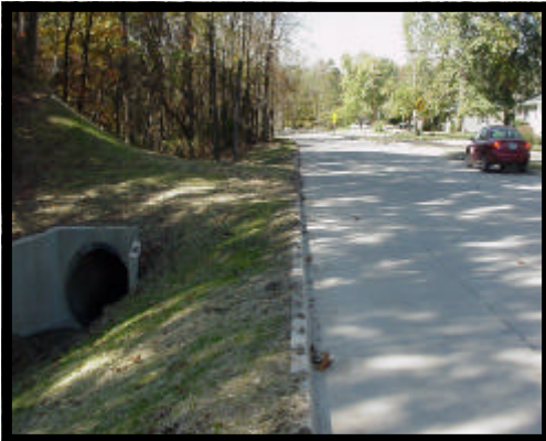
Storm water management culvert for major drainage area adjacent to roadway
