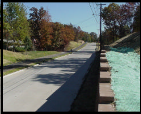
Segmented retaining wall along Beuth Road
