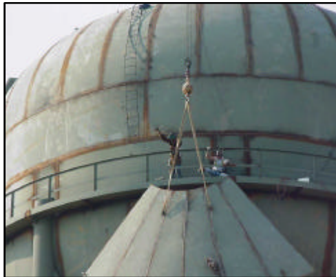
Attaching the top shell of the tank
