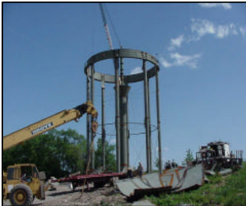
Erection crew at work
