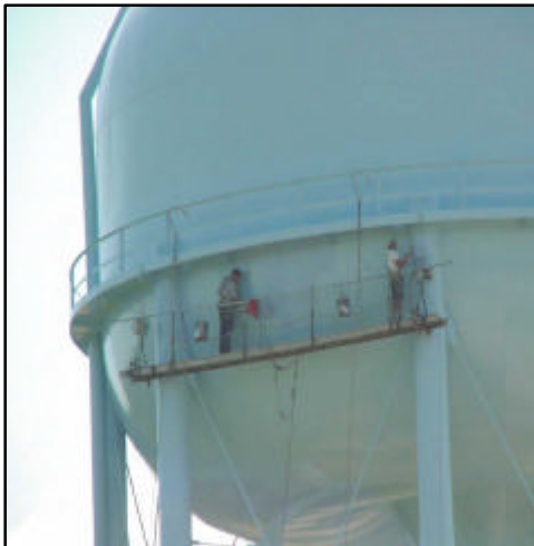
Final coat of paint
