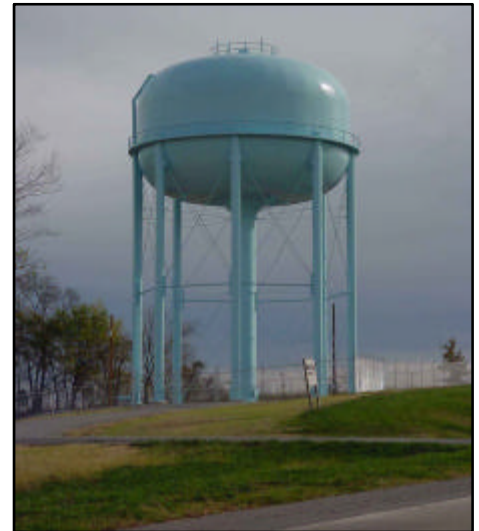
Completed 750,000 gallon elevated tank
