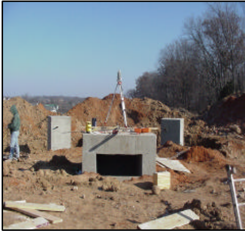
Foundation construction underway
