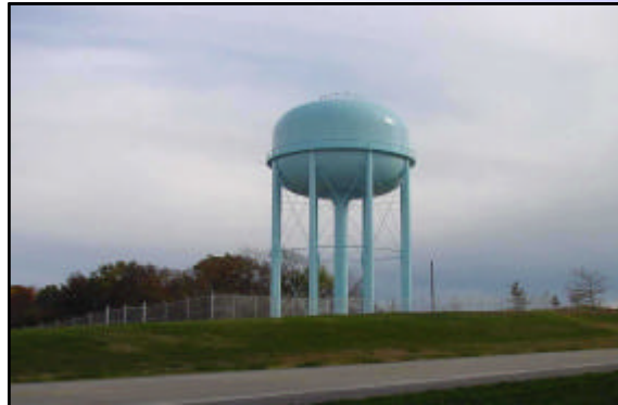
New 750,000 gallon elevated tank
