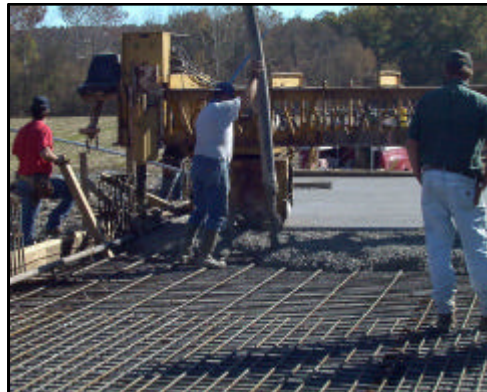
Pouring the concrete deck
