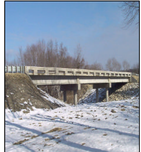
Finished bridge in service
