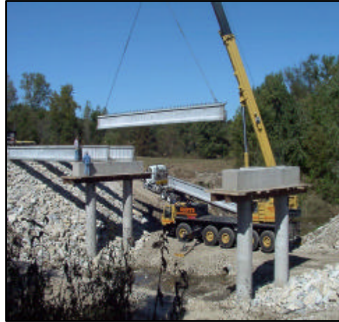
Precast I girders
