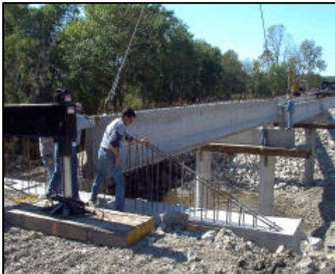
Attaching the girder to abutment
