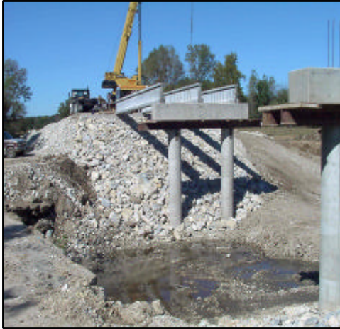
Setting the first set of girders
