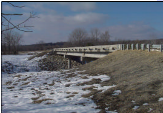
Osage Bridge over Baileys Creek
