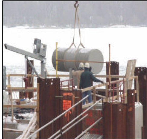
Hoisting filter screen into place
