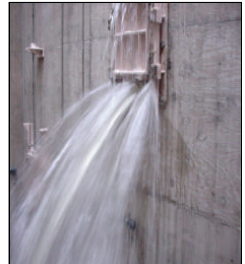
Opening the sluice gate
