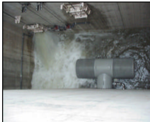
River water being let into the Intake
