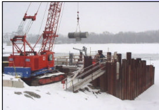
Filter screen hoisted into intake
