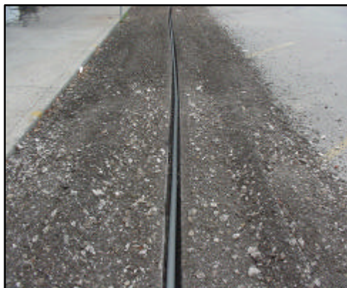
Laying cable Main St. Warrenton MO
