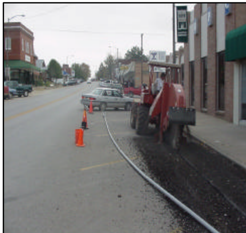
Installing lighting cable Warrenton MO
