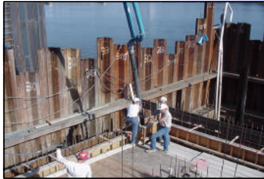
Inside the coffer dam Mississippi River
